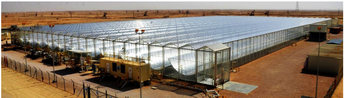
Figure 2: GlassPoint pilot plant, South Oman
