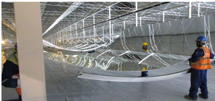
Figure 3: Lightweight mirror installation, 3 workers, no crane, no work at height
